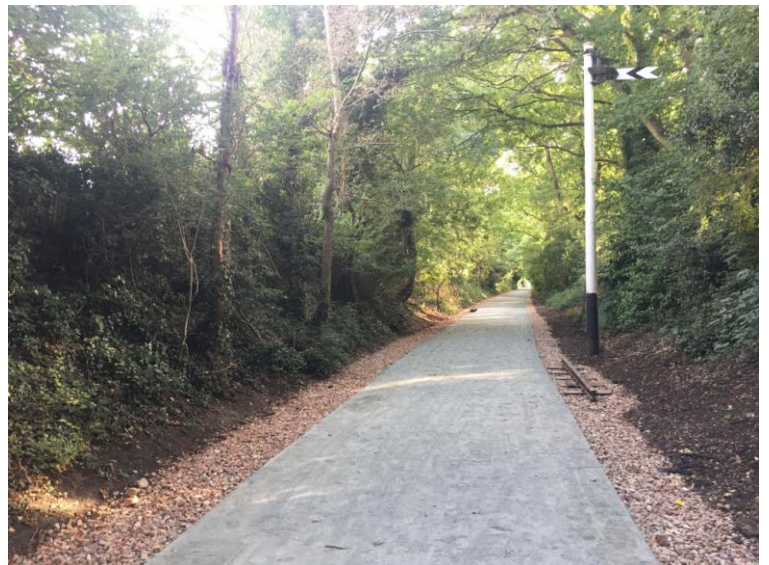
New Crushed Concrete Surface by Roundwood
