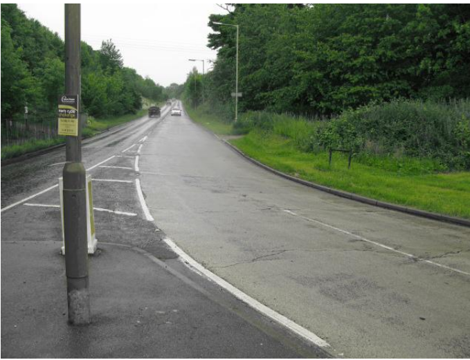
View towards Harpenden from Redbourn Lane Island
