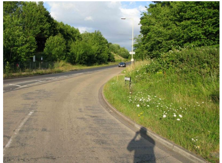
First Clear View towards Harpenden from Car Park Corner – from Middle of First Lane
