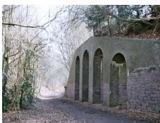
This large brick buttress was built when the tight southward curve was added in this deep cutting so that trains would turn to Harpenden station rather than use the original north curve towards Luton.
